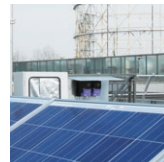
ITALY Cooling loop flow & temperature control
